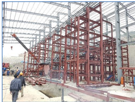
Steel structure rig frame system
