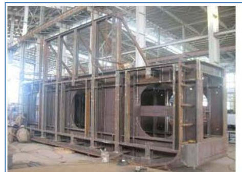
Steel structure (Fender)
