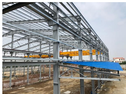
Steel structure erection
