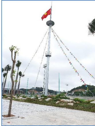
Multi-edge steel column
